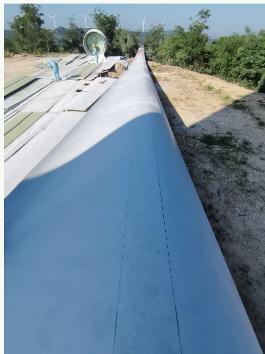
Process of cutting and shredding to recover and repurpose retired wind turbine blades
