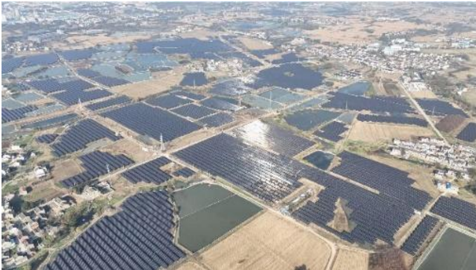
CLP’s Yixing I Solar Power Station in Jiangsu
