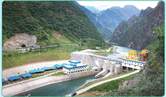
Sichuan Jiangbian Hydro Power Station
