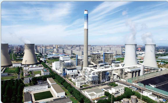
Hebei Sanhe Power Station
